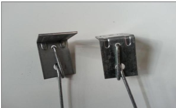
Figure 6. Hanger wires and connection devices
