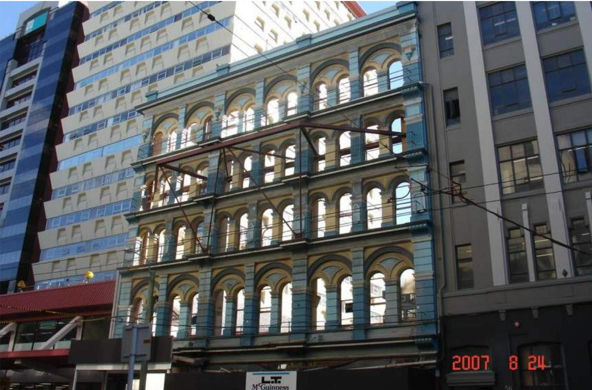
Figure 11: Ballinger Building with temporary facade retention
