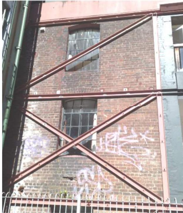
Figure 3: Stiffness incompatibility between strengthening and existing elements
