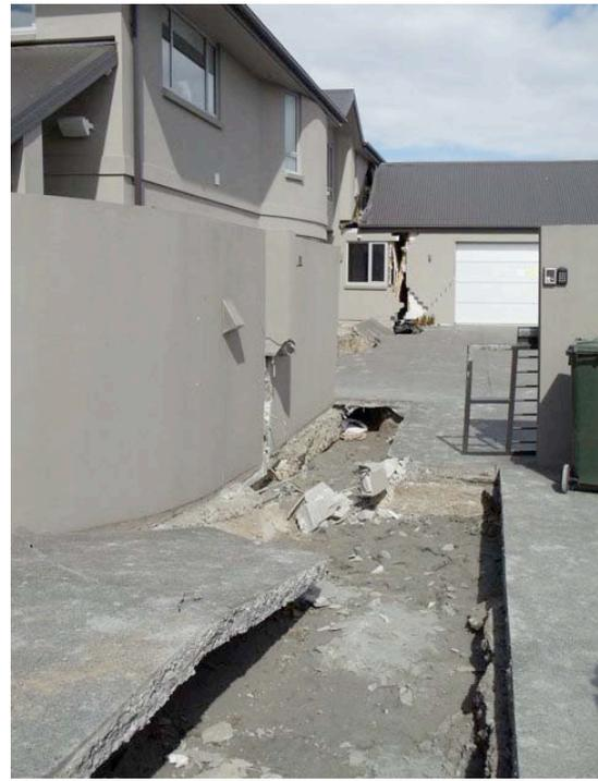
Examples of liquefaction and lateral spreading damage at Kaiapoi NZ (photos by Kevin McCue)
