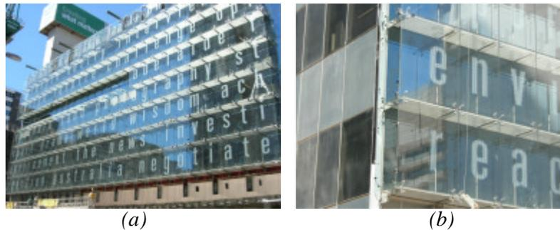
Figure 3 - Building One, butt jointed glass façade supported on “spider” corner fixings
